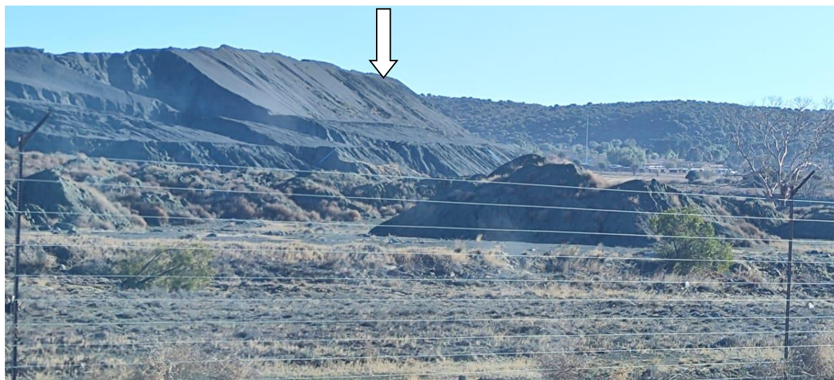
Figure 18 The remaining corner of the Jagersfontein dam wall above Itumeleng
