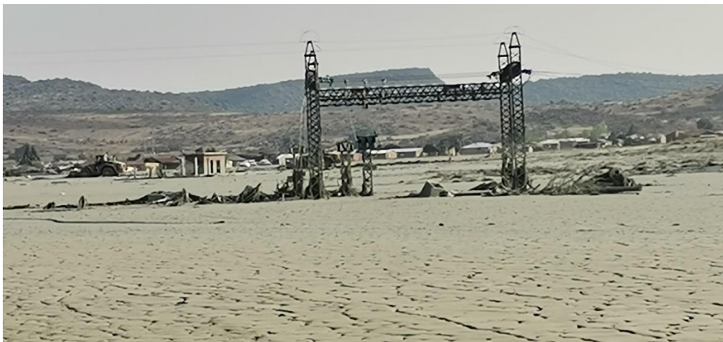
Figure 24 Remains of the electricity substation of Jagersfontein (Photo credit David van Wyk and Brown Motsau)
