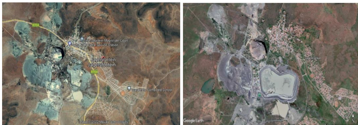
Figure 4 Photos of Jagersfontein tailings in 2005 and 2022 (Google Earth)
