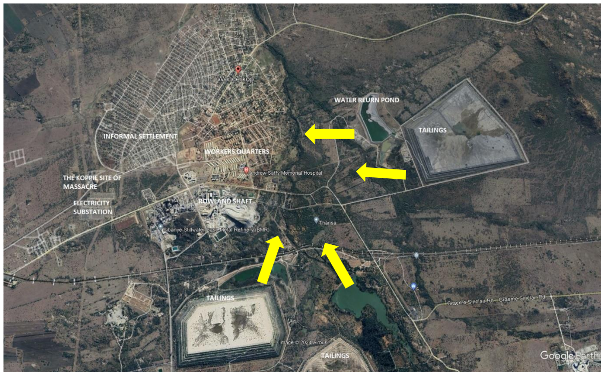
Figure 20: The proximity of major tailings facilities to the Marelwane River located on a sloping elevation above the Wonderkop community (the yellow arrows denote down slope).
