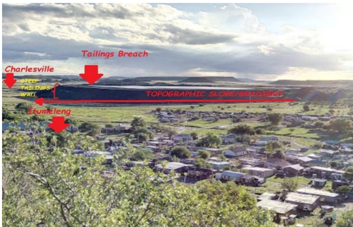
Photo 3 Slope, gradient of tailings and location of the two townships from a vantage point to the north (Adapted from Google Maps)
