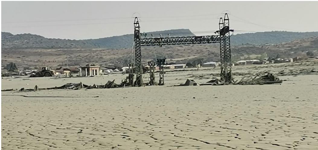
Photo 6 Remains of the electricity substation of Jagersfontein (Photo credit David van Wyk and Brown Motsau)
