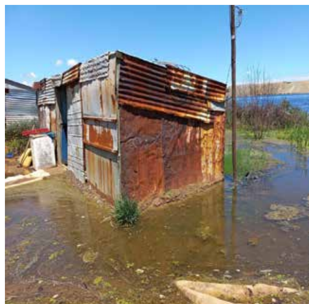
Flooded house in Nyakallong
