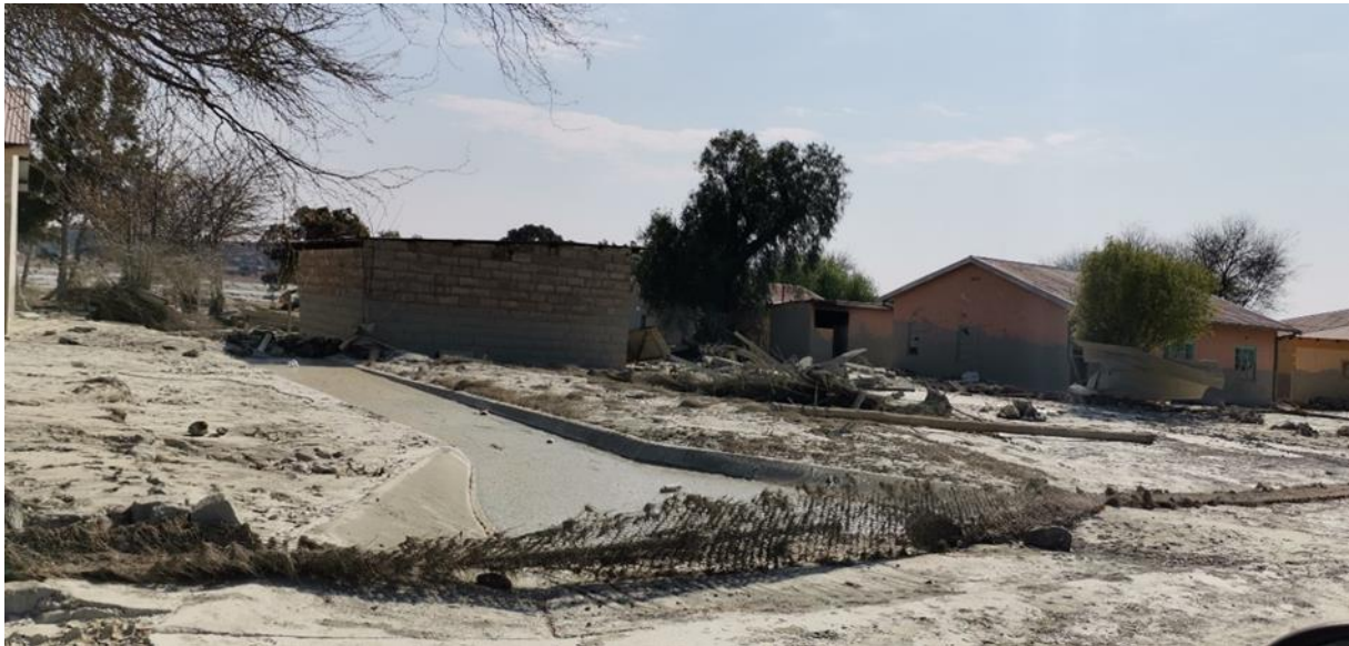
Figure 7 The only thing left of these Charlesville houses in the front of the photo are their foundations (Photo Brown Motsau and David van Wyk)
