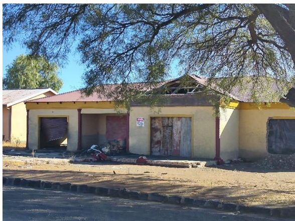
Figure 9 A disaster-damaged house in the process of being repaired
