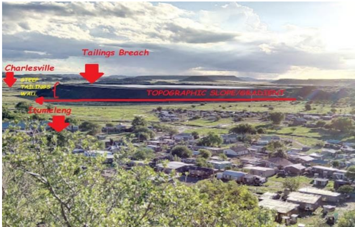
Figure 23 Annotated photograph showing the slope and gradient of the tailings and the location of the two townships (Adapted from Google Maps)
